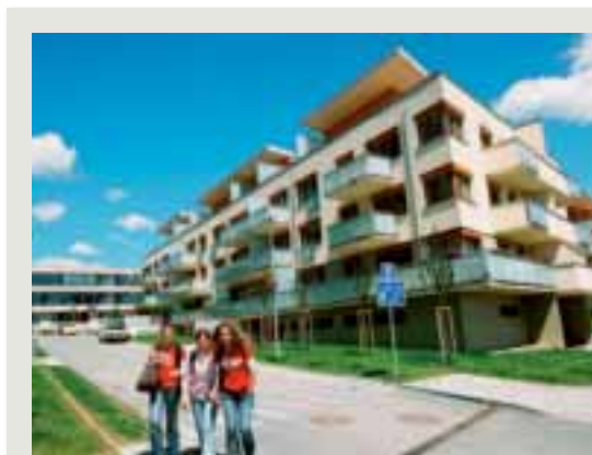
Skanska was responsible for the land purchase, planning, design, construction and sale of the Botanica residential district in Prague.
