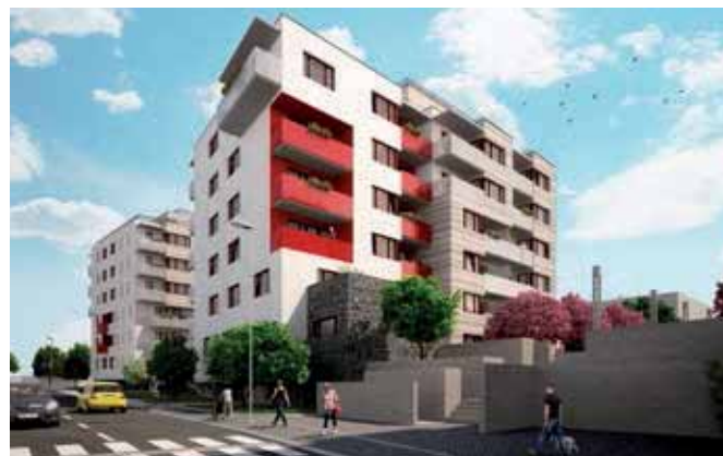
At Botanica K, treated water from washbasins, bathtubs and showers is used for flushing toilets, helping save water and energy.
