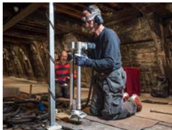
Sandvik has replaced 4,000 rusty bolts on the 17th century Vasa war ship at the Vasa museum in Sweden.
