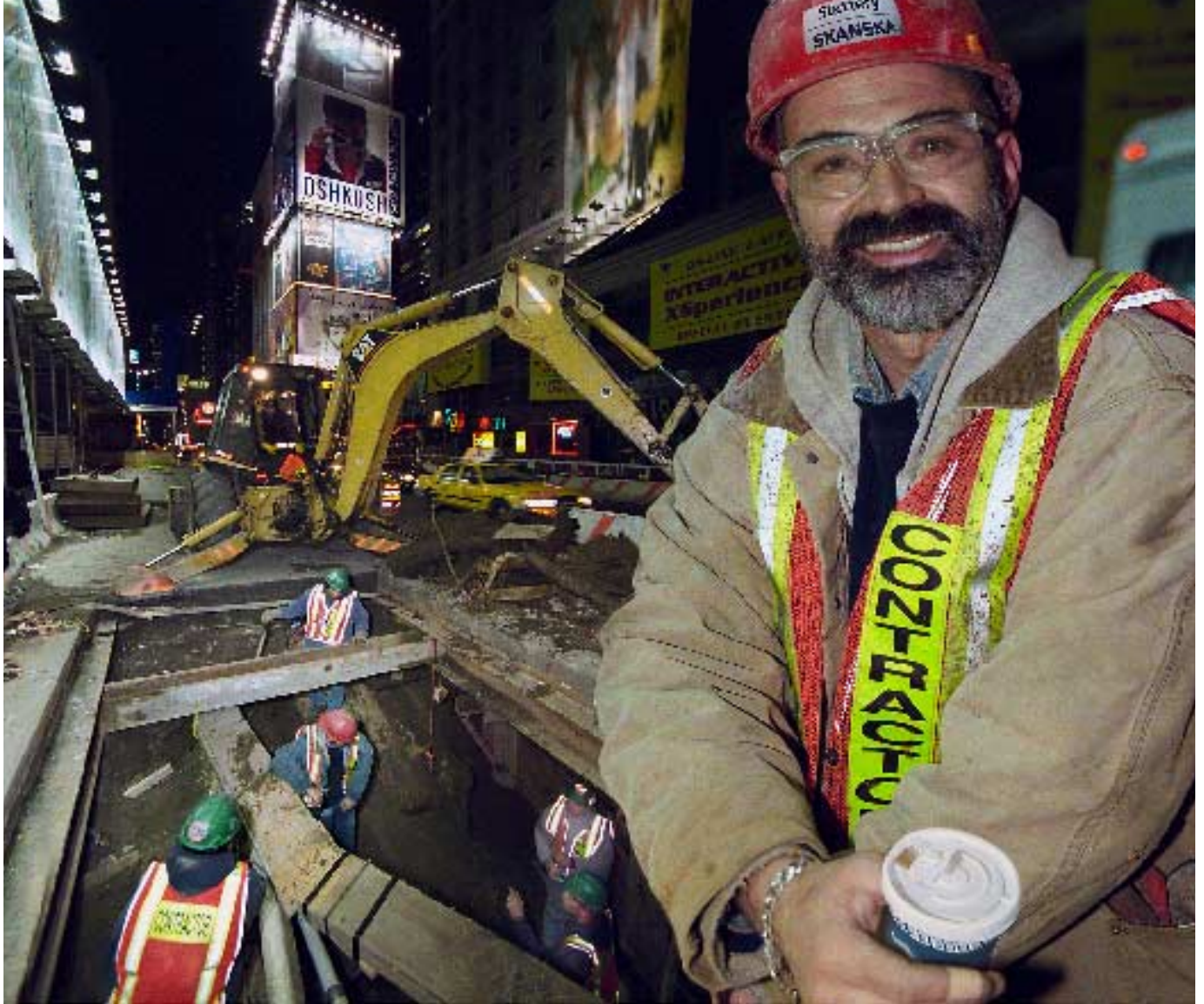
Jesus Mangual heads a work crew at Skanska Slattery, which is a participating contractor in the extensive modernization of the Times Square subway station in New York. In order to cause as little disruption to Manhattan's hectic traffic as possible, most of the work is done at night.
